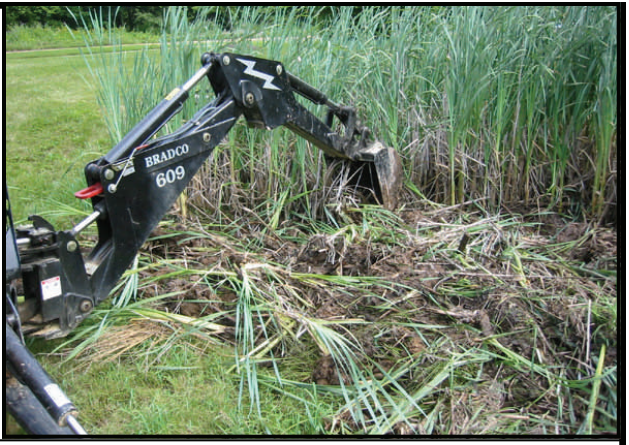
During construction, cattails were completely removed from the basin, allowing for native vegetation to establish in the wetland.
