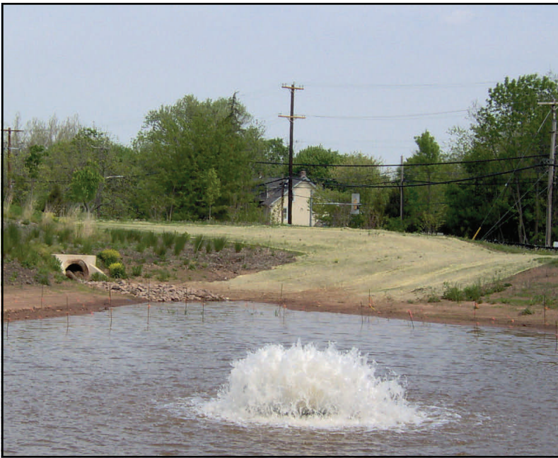
Above: An aerator promotes water quality by adding dissolved oxygen to sustain plant and animal life. Aerators are necessary in any wetpond that does not have lowing water input.
