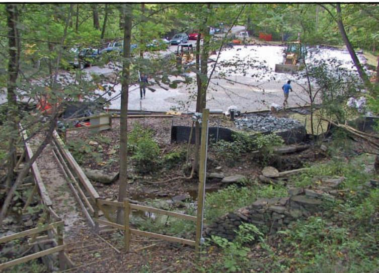
The BMPs at Riverbend help control stormwater runoff into Saw Mill Run, near its confluence with the Schuylkill River. First, water will infiltrate through porous pavement and then discharge through a “bio-swale” where wetland plants further filter the outflow before it discharges into Saw Mill Run. The process of plants’ evapo-transpiration will also help reduce the volume of storm water.
